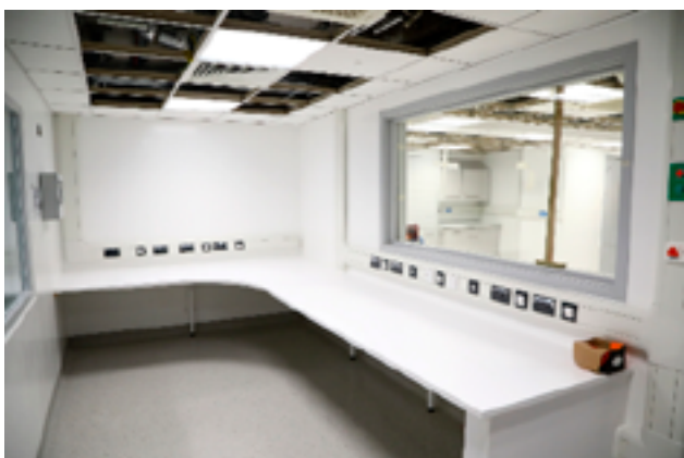
Internal refurbishment to create a CT scanning area
