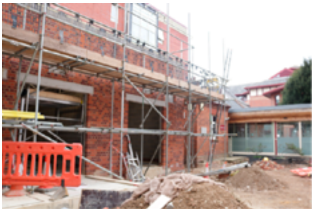
Work progressing on the creation of an electrical substation
