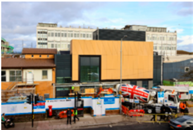
External shot of the Emergency Department progress
