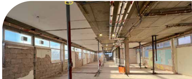
Internal strip out at the Cauldwell Centre is underway
